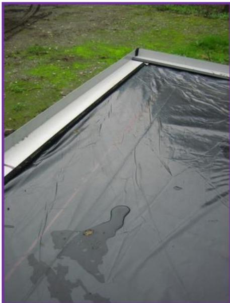
*Metal edging attached with 5mm thick adhesive pads*
